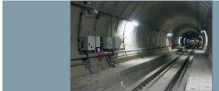
TGV tunnel in Belgium
